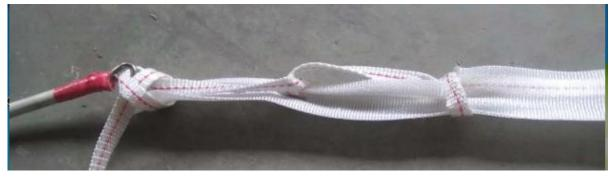
b) Use a pull tape of about 1m long to make a fast knot on the 3cm opening. Then make 2-4 half knots
