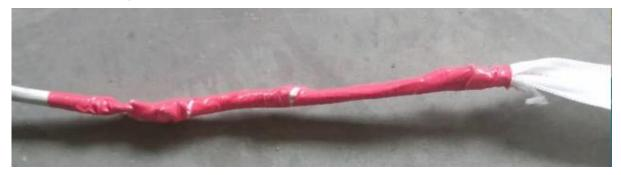
c) Overlap three inner ducts for 80cm and cut an opening, and pull out the pull tape of one of inner ducts to make a fast knot and then make 2-3 half-knots for tensioning.
